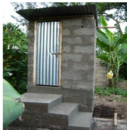
Fig. 6: Concrete block single vault UDDT in Daraja II (Source: ROSA).
